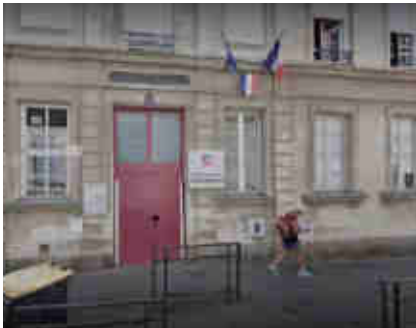
Nursery School Parcheminerie (France)
