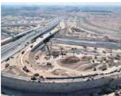
Al Khor Expressway (Qatar)
