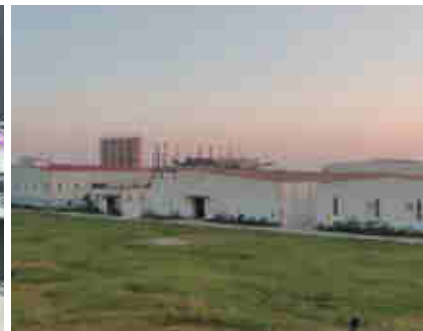
Akij Plastics Chhatak Plant (Bangladesh)
